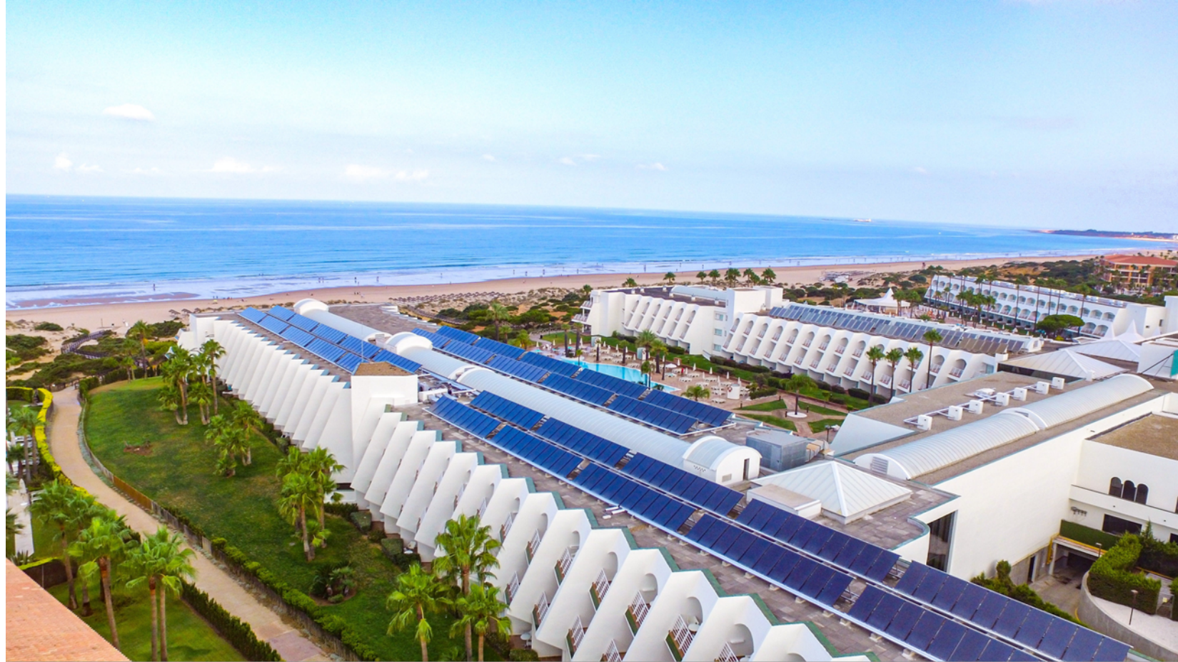
Hybrid solar – PVT installation on hotel roof, Spain.
