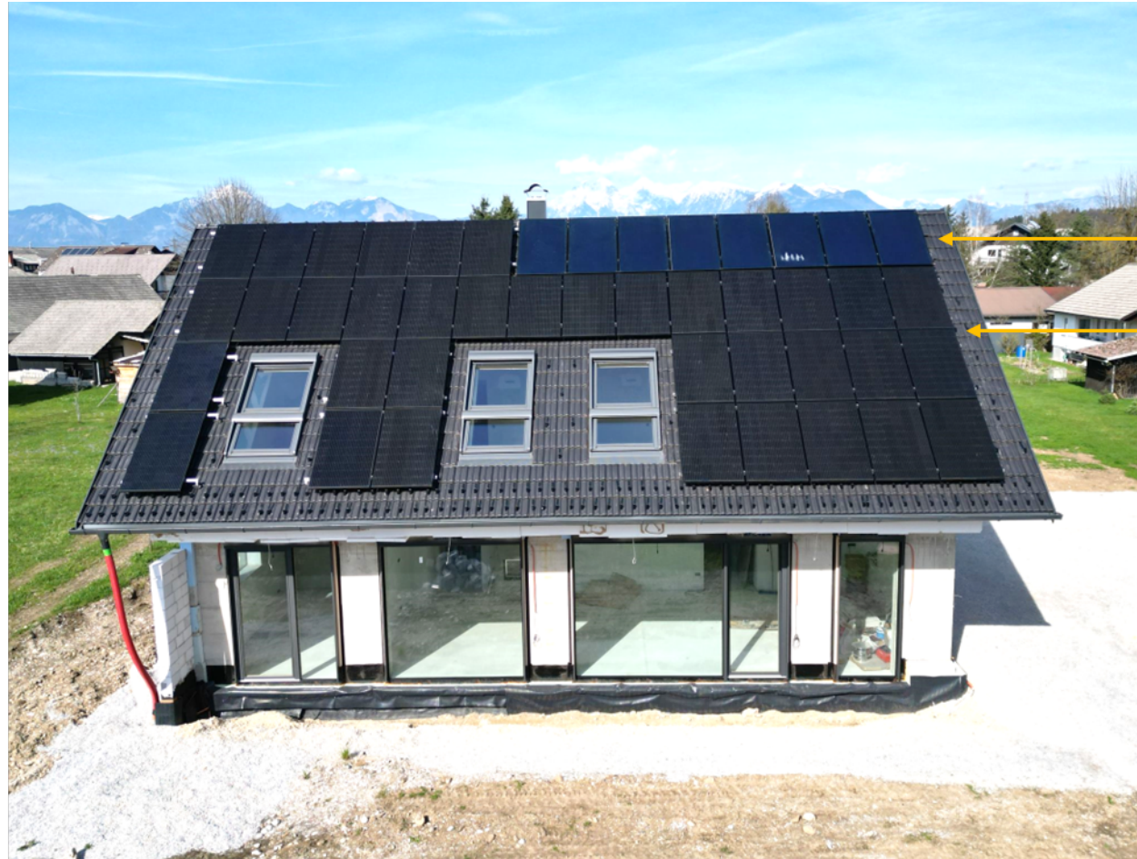
Solar thermal and solar photovoltaic sharing the roof of residential building, Slovenia
