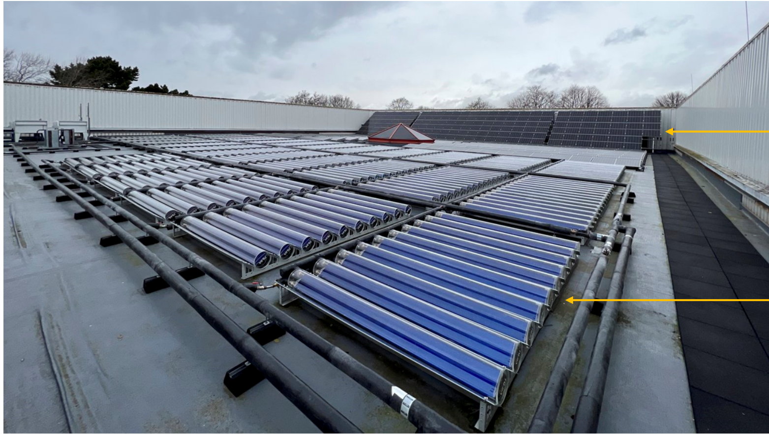
Solar thermal and solar photovoltaic sharing the roof of a leisure centre, Southeast England
