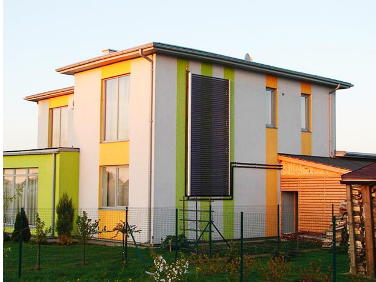
Solar thermal façade mounting for hot water and space heating on single-family house, Germany
