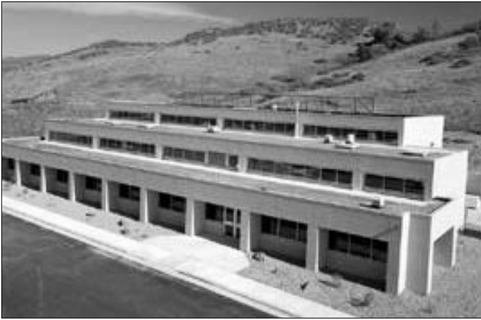
NREL's Thermal Test Facility in Golden, Colorado
