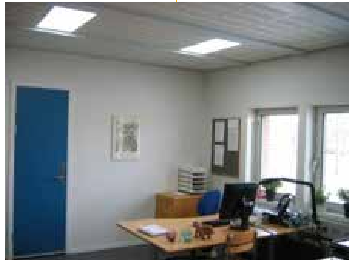
▲ Figure 2. Office with original luminaires with 2700K T8-fluorescent tubes (left). The same office with the new 5500-6000K LED panels (right).
