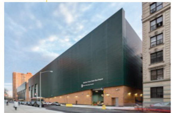
Dark Green SolarWall on the three walls of Bus garage in New York City (Source: SolarWall)
