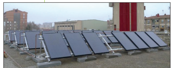
▲ Figure 4. In Spain, 28 PVT glazed panels covering 46 m 2 generates 6.7 kWp for DHW in a firehouse. Electricity is for self-consumption and the grid. (Credit: Endef Engineering)
