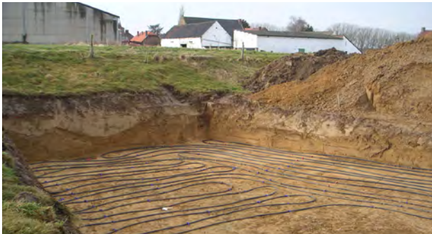
↑ Illustration 260 : Implementation of horizontal collectors.
