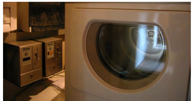
↓ Illustration 56: Provelo renovation: work on the collective laundry room
