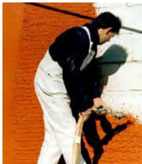
↑ Illustration 172: External coating on masonry
