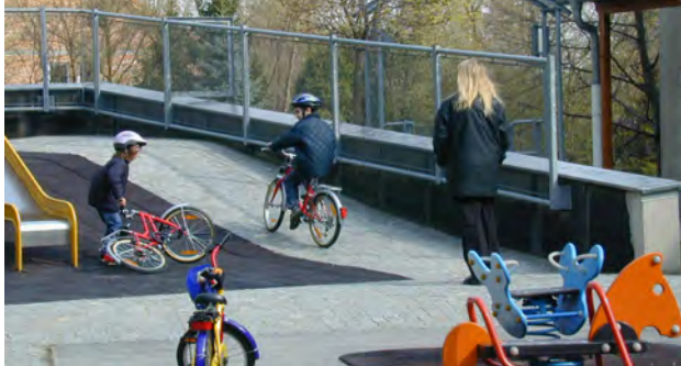
↑ Illustration 60: Brunner housing: work on playgrounds
