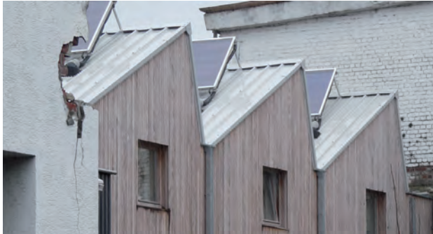
↑ Illustration 278 : Plane collectors in superposition of roof.
