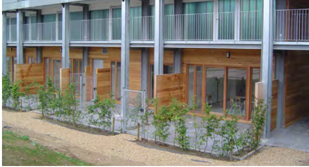
↑ Illustration 58: Sterrenvel renovation : work on private and collective spaces
