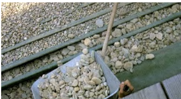
↑ Illustration 372 : Installation of gravel layer
