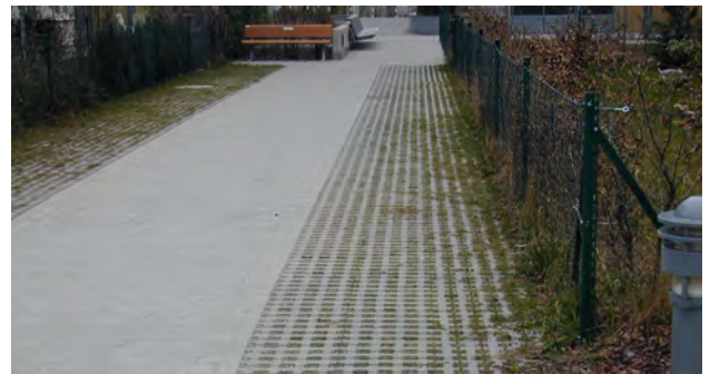
↑ Illustration 361 : Hedge and various coverings to infiltrate rainwater
