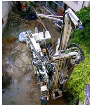
↑ Illustration 261 : Implementation of geothermic pump - vertical collectors.
