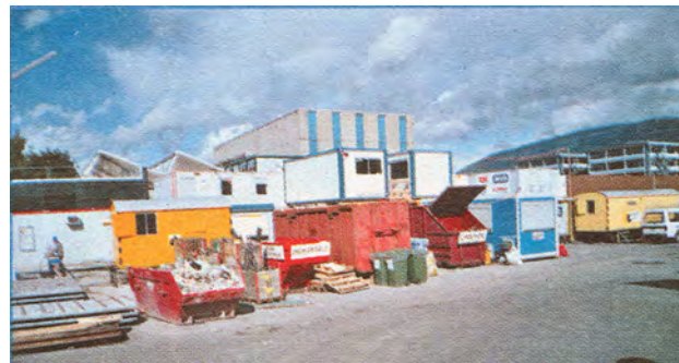
↑ Illustration 389 : Construction waste sorting on building site
