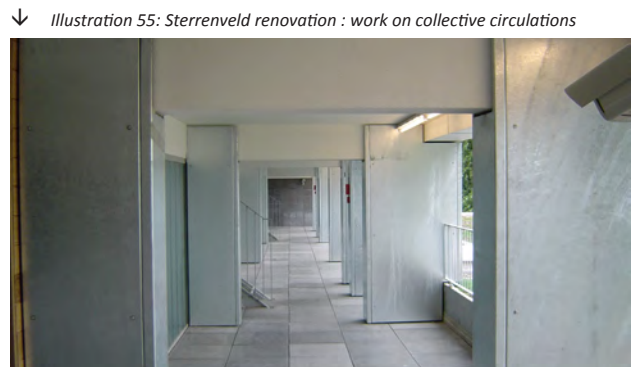
↓ Illustration 55: Sterrenveld renovation : work on collective circulations
