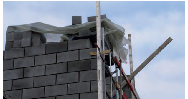
↑ Illustration 421 : Masonry work
