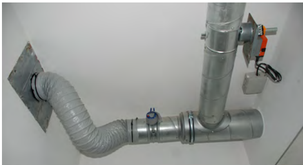
↑ Illustration 90: Installation of a ventilation system - pipes
