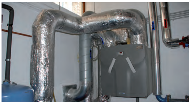
↑ Illustration 225 : Heat recovering - Balance ventilation system.
