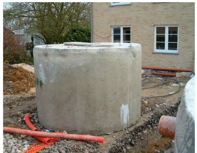
↑ Illustration 347 : Concrete water tank
