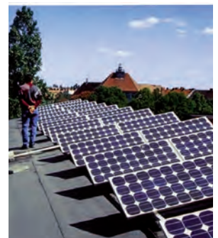
↑ Illustration 319: Installation on a flat roof
