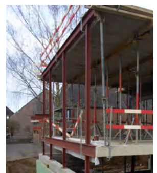
↑ Illustration 45: Steel frame work
