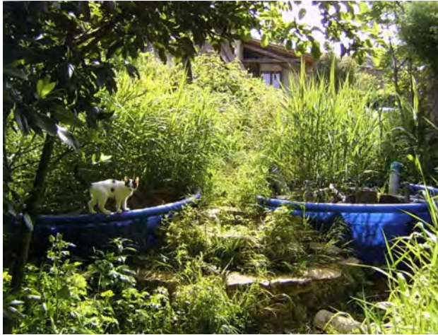
↑ Illustration 371 : Two basins in parallel with a vertical flow
