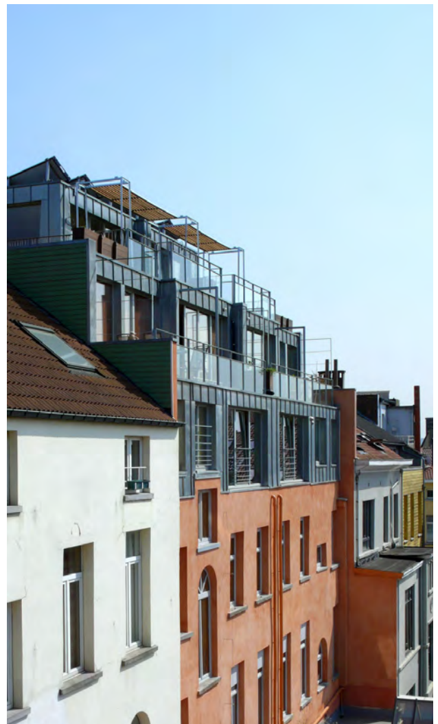
↑ Illustration 53: Housing and offices renovation: 3 housing storeys added in wood frame
