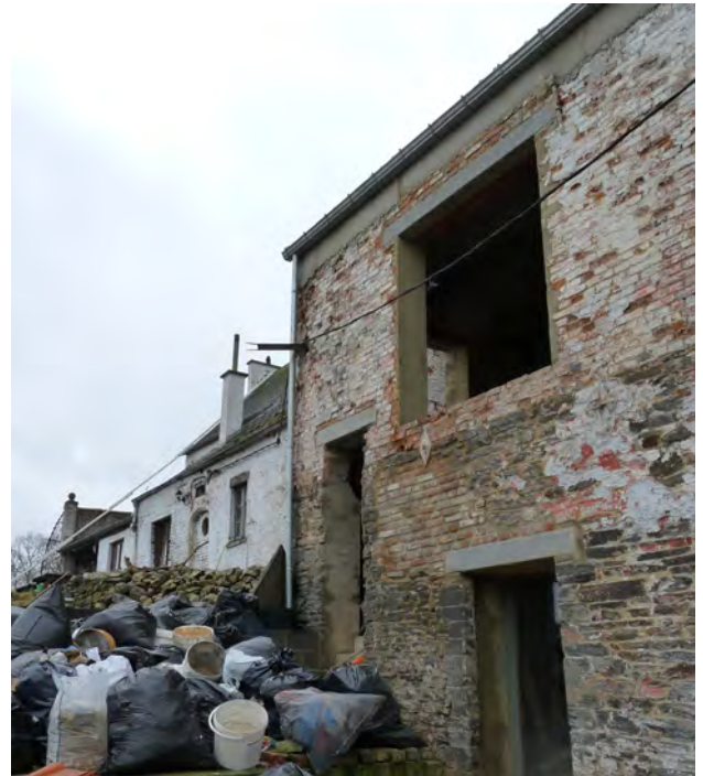
↑ Illustration 50 : Exemple of a large renovation
