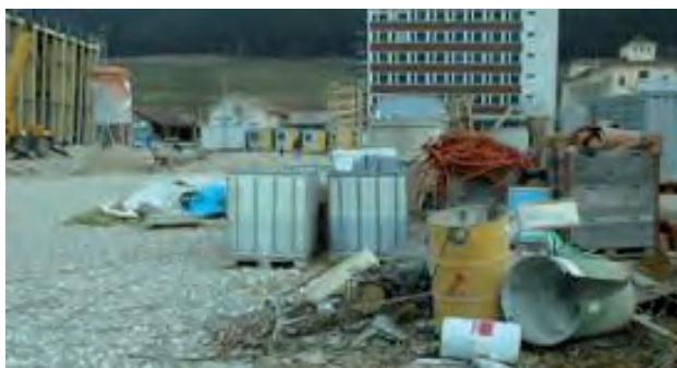
↑ Illustration 418: Production of waste on building site
