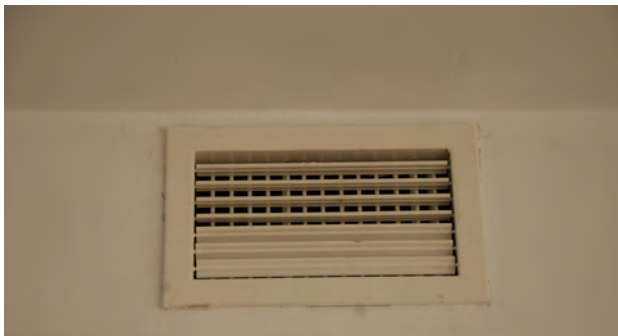
↑ Illustration 91: Installation of a ventilation system - grille
