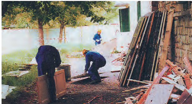
↑ Illustration 398 : Wood waste sorting on building site
