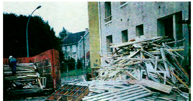
↑ Illustration 22: Sorting out the construction waste: container with wood
