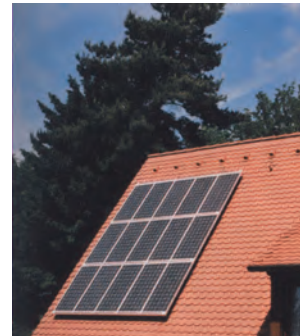
↑ Illustration 318: Installation on a roof
