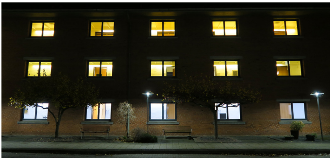
Figure 2. Exterior night view of Vikaergaarden rehabilitation facility with existing fluorescent lighting (two top floors) and new dynamic LED lighting (bottom floor).
