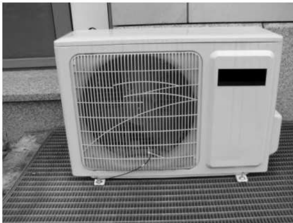
Figure 10: Installation of budget Mono-split-unit at ILK Dresden [EvaSolK 2013]
