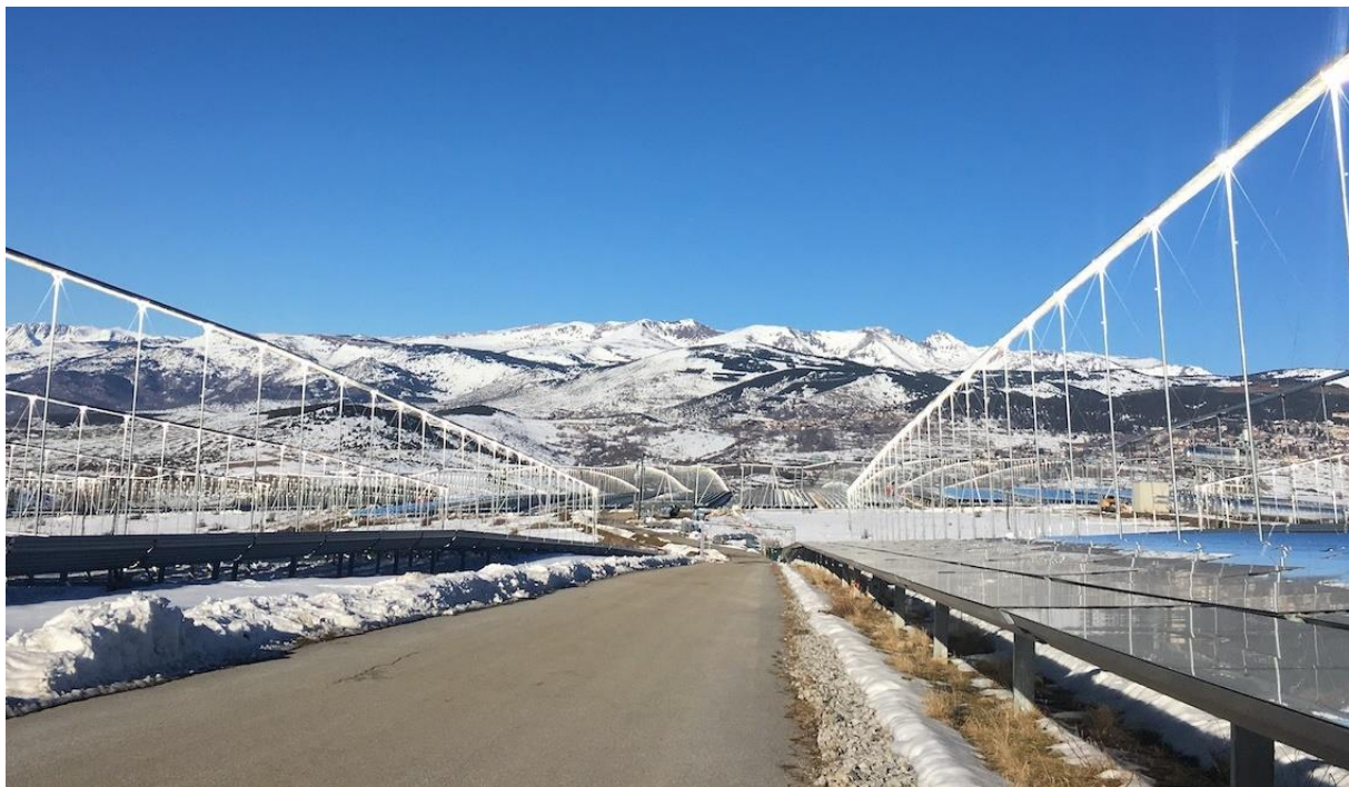
Figure 22 Photo of linear Fresnel collectors Ello Module, Ello (manufacturer information)
