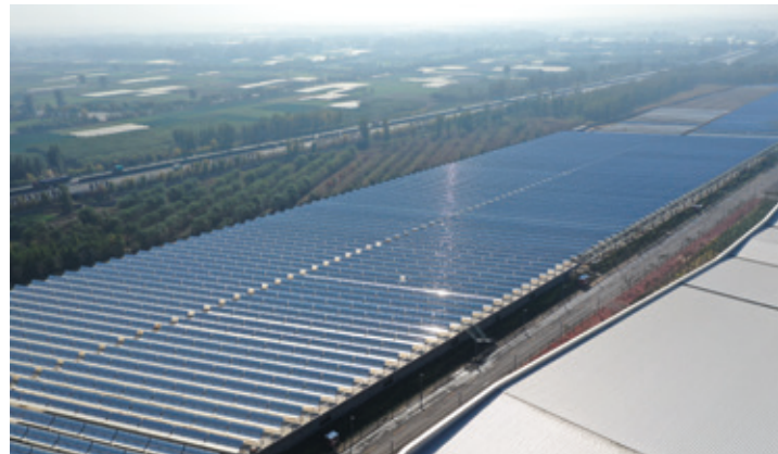
An 80 MW th parabolic trough collector system supplies snow for an indoor ski hall, as well as heating and cooling at the Handan Bay Water World in China
