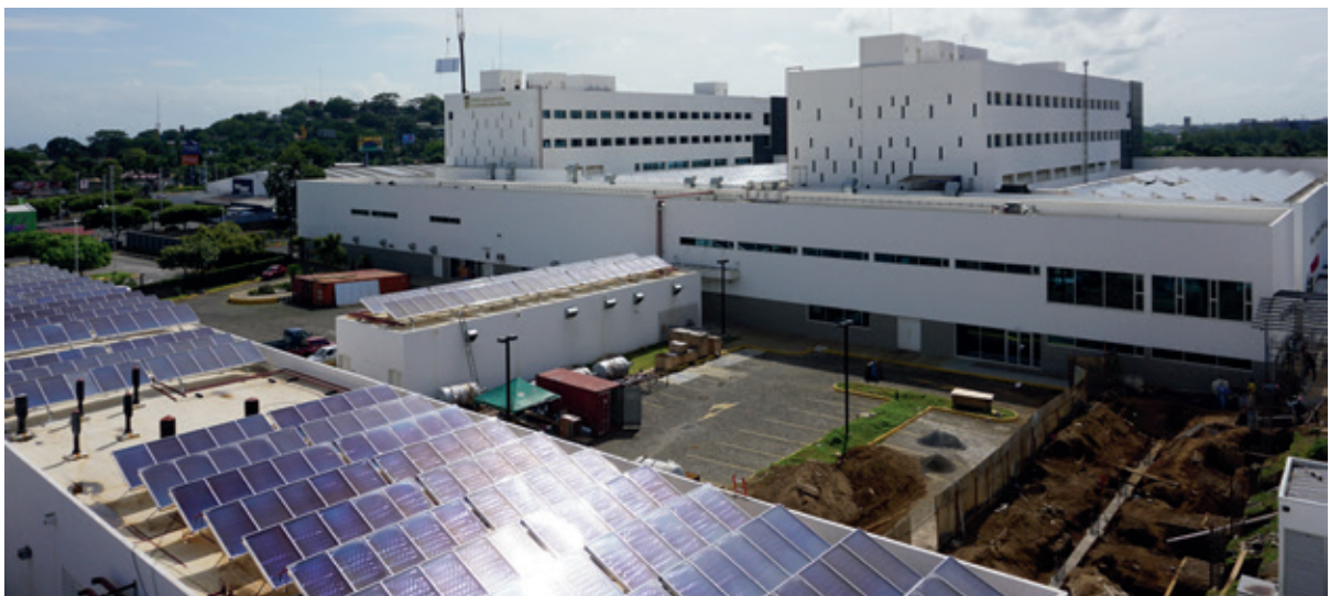
1 MW Solar cooling system at the Hospital Militar Escuela in Managua, Nicaragua
