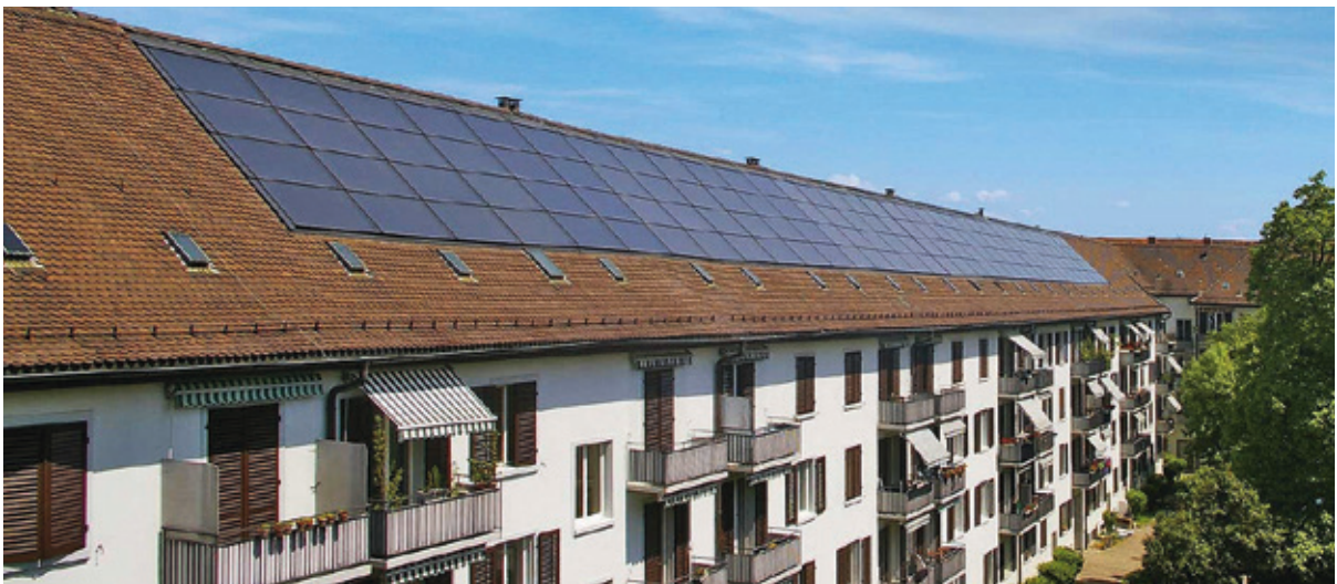
Solar thermal system for an apartment building in Zurich, Switzerland
