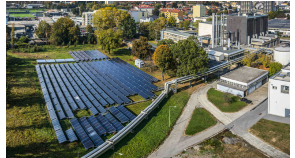
Test field with large collectors on the former dump site beside the DH plant in Graz
