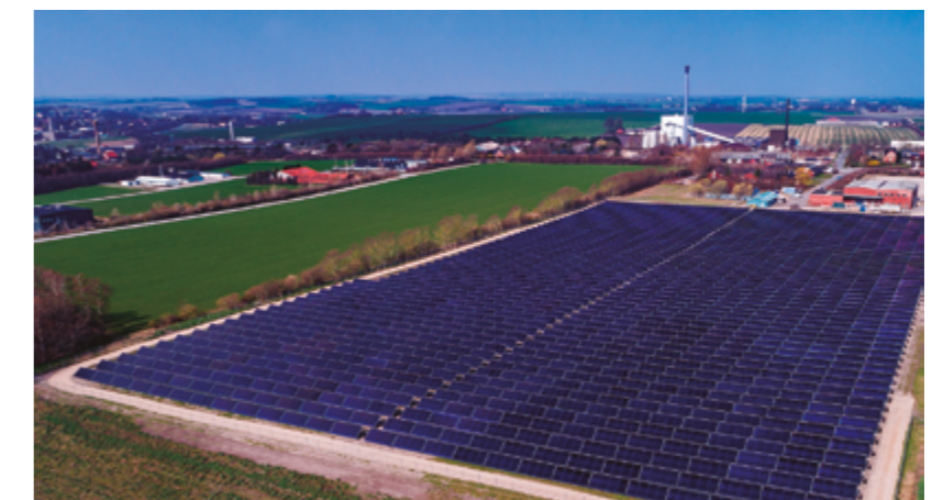
14.5 MW collector field intalled on a former industrial site PHOTO: SAVOSOLAR
