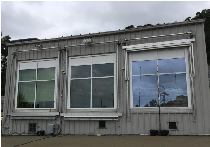
Figure 6. Outdoor view of the roller shade, auto-GG shade, and Venetian blind (from left to right) in the LBNL Advanced Windows Testbed, Berkeley, California.
