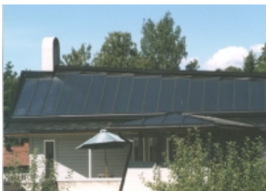
Fig. 8 Single-family house, Oslo, (solar combisystem; collector area: 30 m 2 , storage volume: 3 m 3 )
