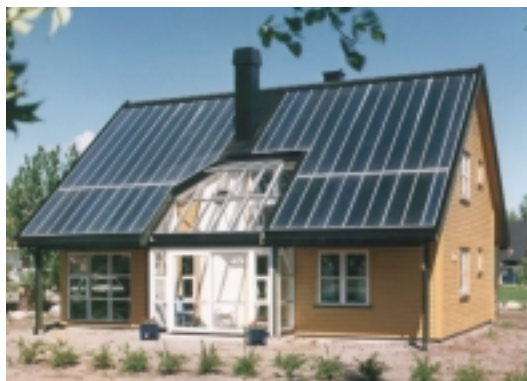
Fig. 7 "April house" in Tønsberg, Norway (solar combisystem; collector area: 20 m 2 , storage volume: 1 m 3 )
