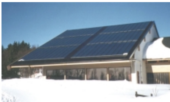
Fig. 6. Ranten Mountain Resort, Nesbyen, Norway (solar combisystem for DHW-, space- and swimming pool heating; collector area: 200 m 2 , storage volume: 4 m 3 , pool volume: 90 m 3 )
