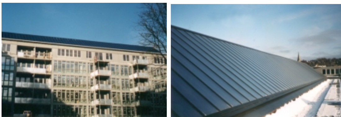
Fig. 1: The Klosterenga residence in Oslo with a solar combisystem, 218 m 2 collector area.
