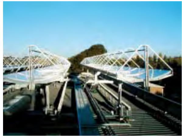
300 m 2 Bruce Hall system under construction
