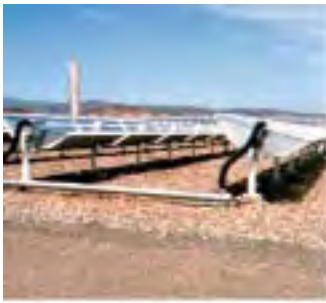
Fig. 18: Troughs can be connected in series and/or in parallel to form a larger collector array (picture source: AEE INTEC, Austria and CIEMAT, Spain)
