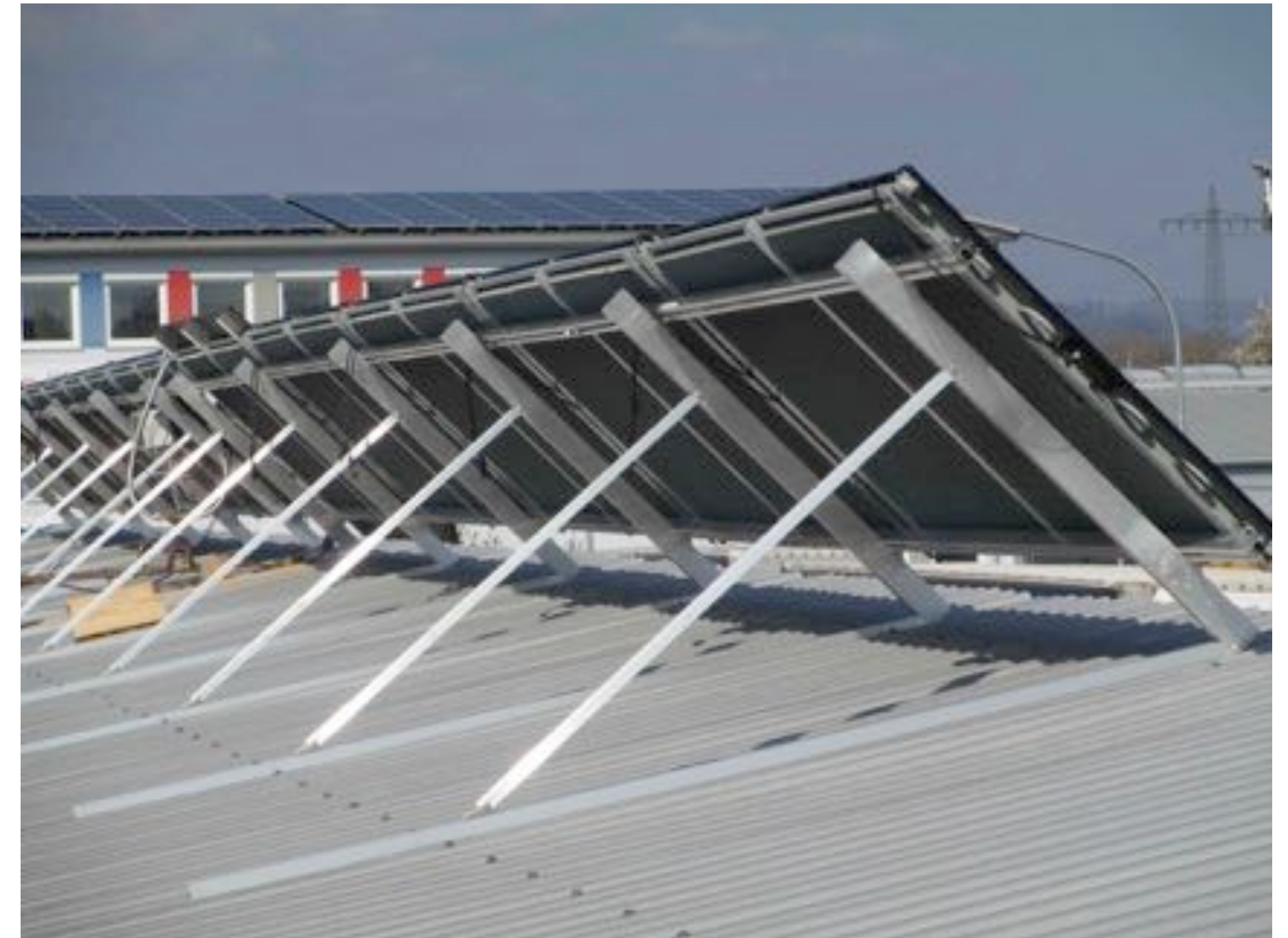
Consolar building, Lörrach
